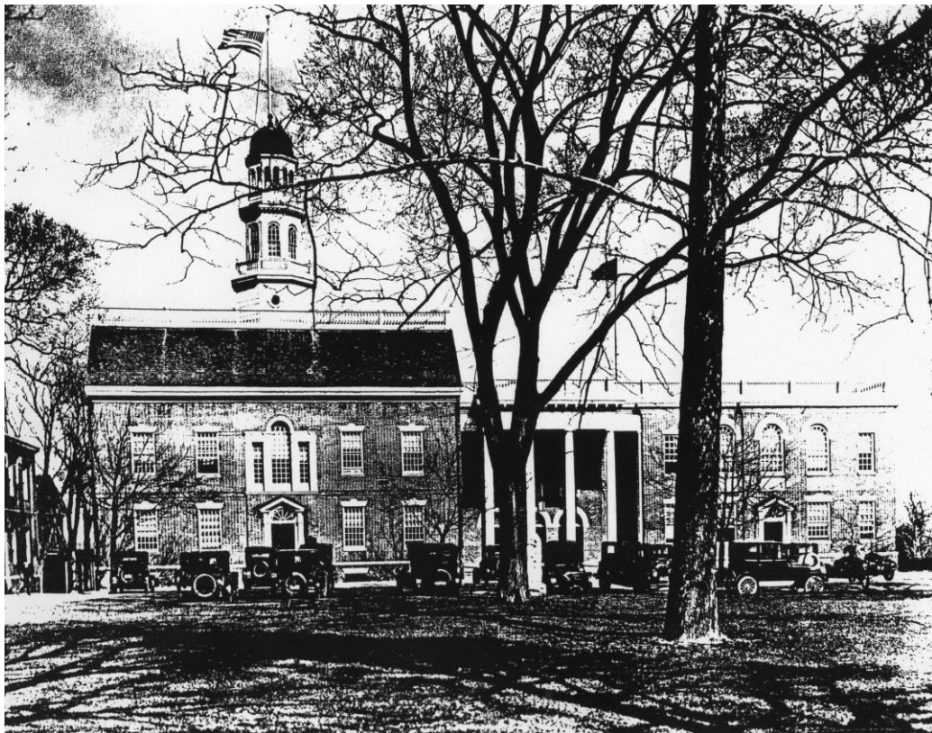
Figure 2-5: Photograph Showing the 1906 Renovations (from Wise 1978).
