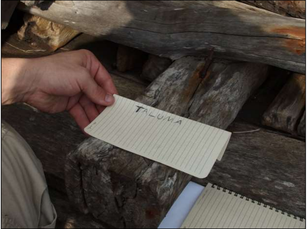
Author indicating the taluma , or alternating Y-frame, Tongoni Village, Tanga Region (Photograph by Madeline Roth)
