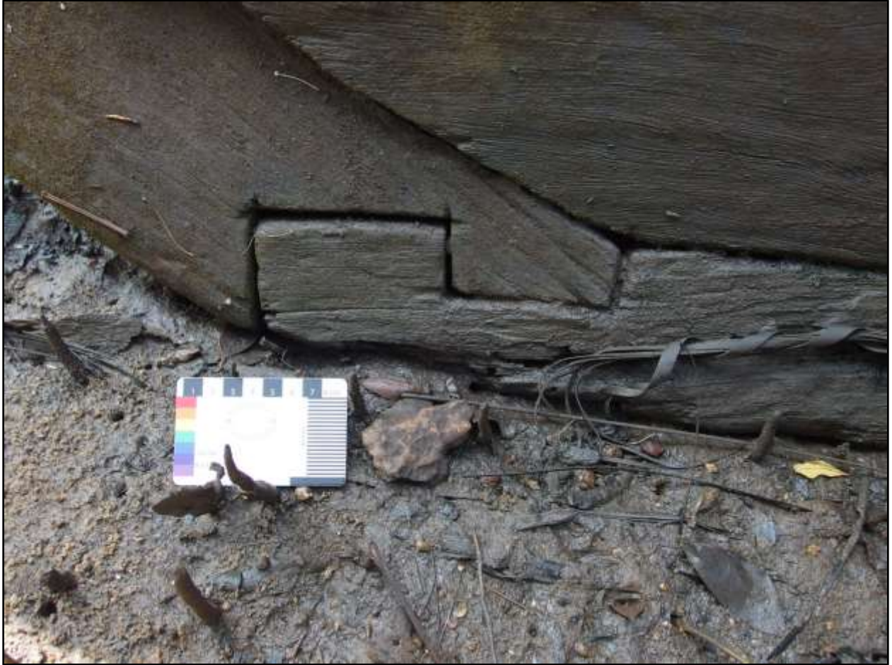
Scaled photograph of the kufuri joint, Tongoni Village, Tanga Region (Photograph by Madeline Roth)
