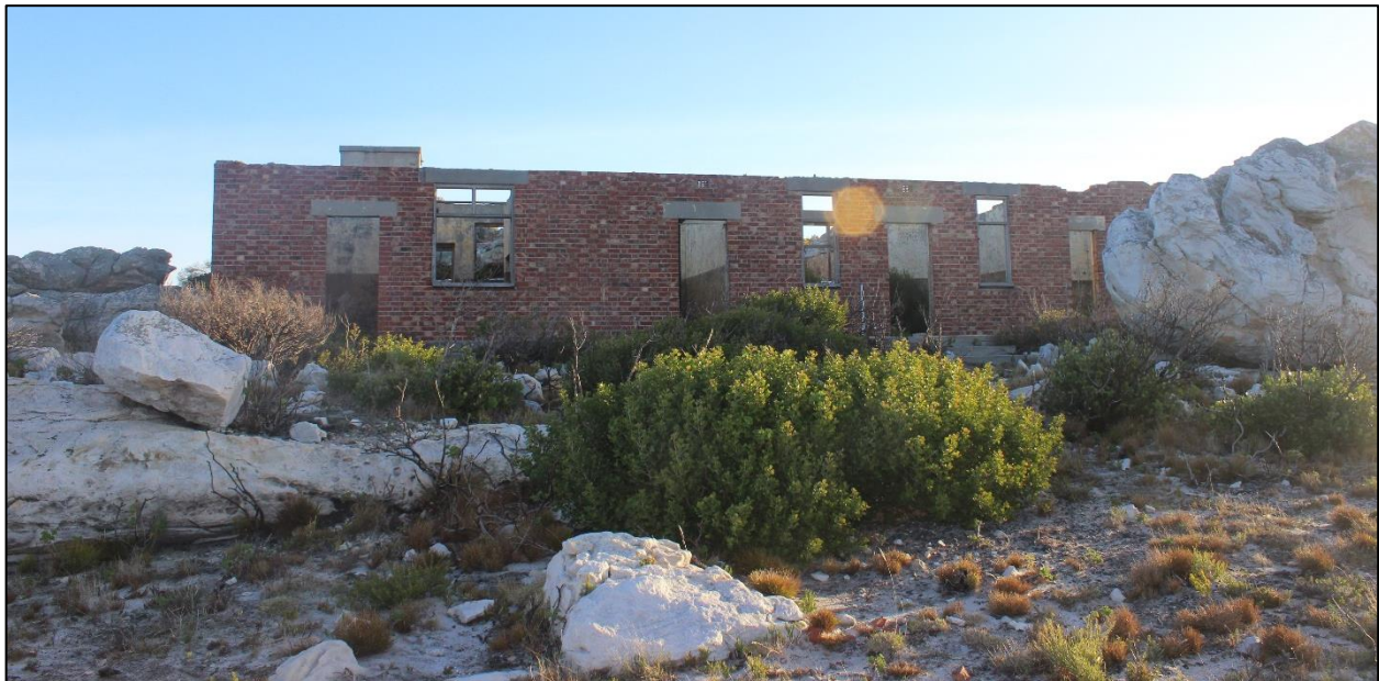
Figure 18: Photo of the main dormitory structure at the Olifantsbos RDF Station, Cape Point National Park, Western Cape RSA. Poking out from above the dormitory on the left side is the square cement RDF equipment case or cistern Photo by author, 2017.
