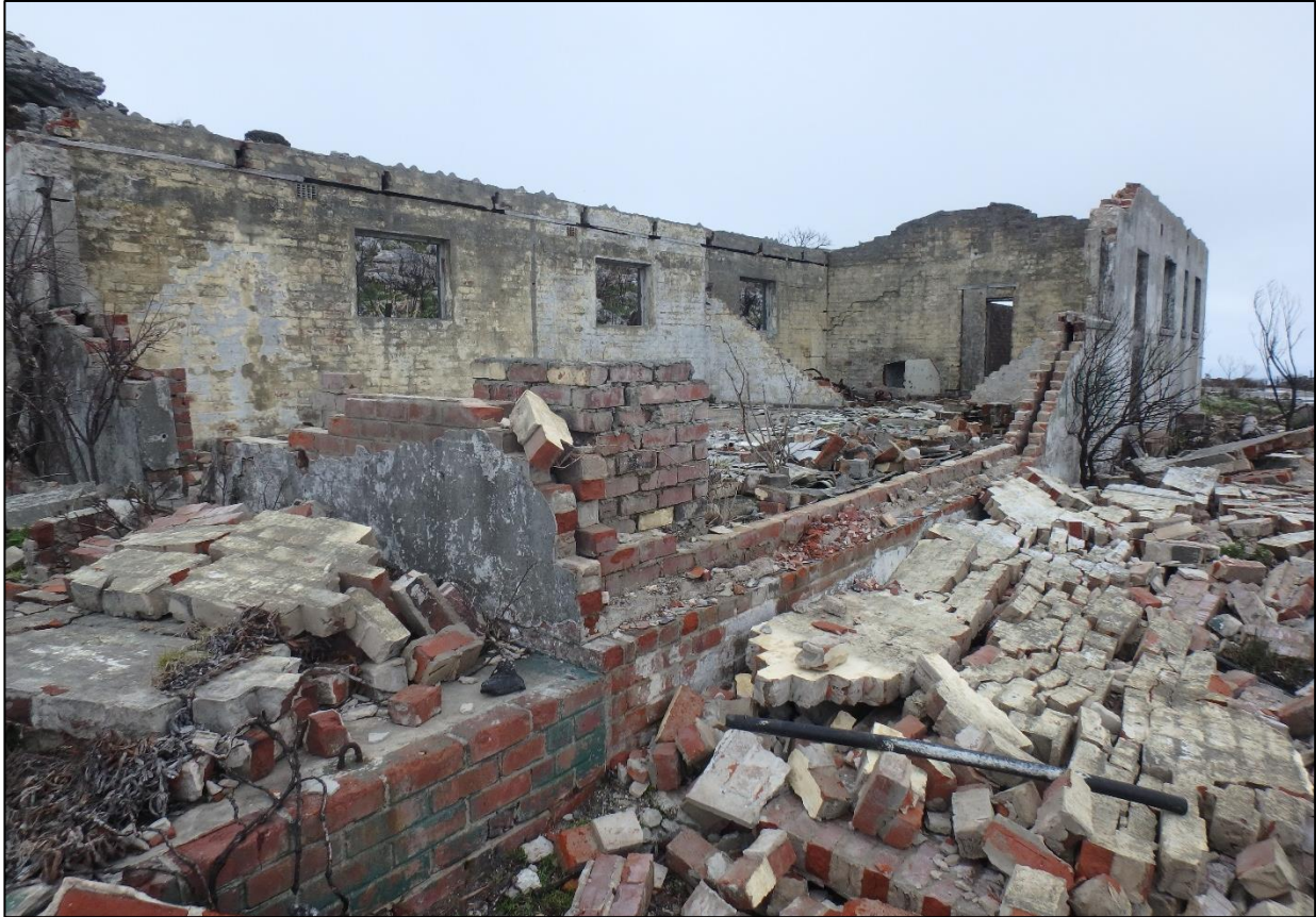
Figure 14: Photo of the Main Dormitory building at the Karbonkelberg RDF station. Photo by author, 2017.
