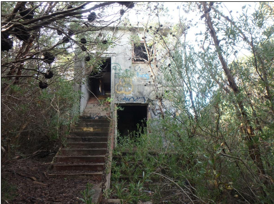
Figure 12: Image of the rear face of the Glencairn Hill Battery Observation Post. Unique for its two-story design. Image by author, 2017.
