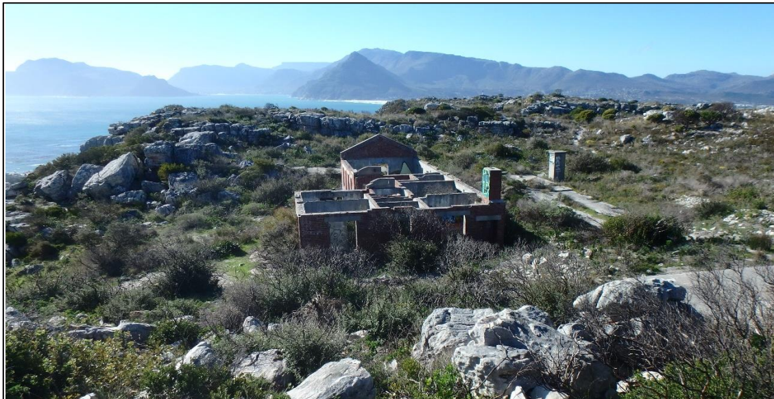
Figure 24: Photo of the main dormitory structure, Slangkop RDF Station, Western Cape RSA. Image by author, 2017.
