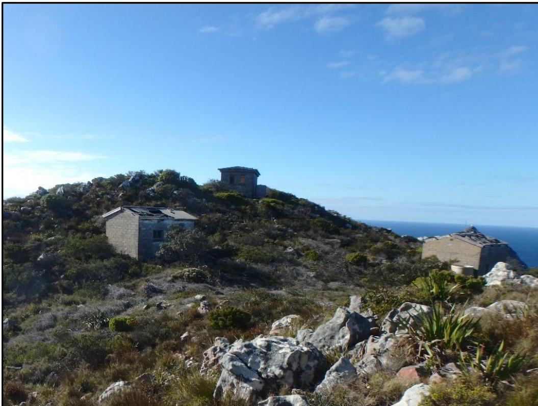
Figure 20: Photo of the Rooikrans RDF station upper site. Structures: 908 Building (left), main operations building (center), and wash-house (right). Image by author, 2017.
