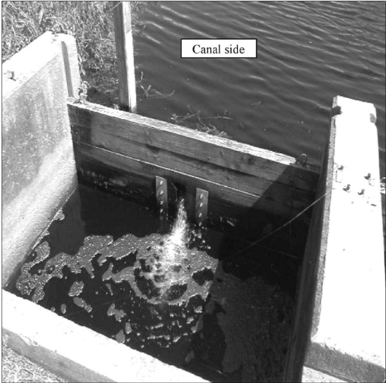
Figure 1.4. Photograph of one of the fish passage slotted weirs that were installed in 1996 in existing wooden stop blocks in an effort to enhance fish and blue crab passage (Rulifson and Wall 2006).
