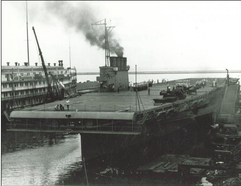
Figure 2.6. Finishing conversion of USS Wolverine , August 1942. SS Greater Buffalo , left, is ready for conversion into USS Sable . (Courtesy, National Museum of Naval Aviation).
