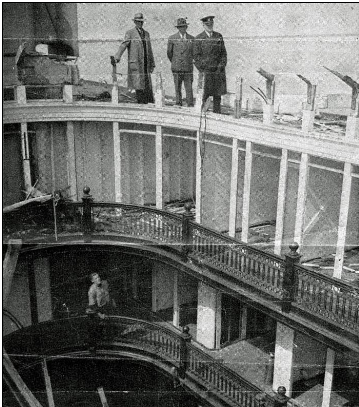
Figure 2.2. SS Seeandbee 's fancy staterooms and atrium being stripped down. (Scharch, Ed L., "USS Wolverine (IX-64) WWII Training Carrier 1942-45," http://www.scharch.org/Ed_Scharch/23-uss-wolvering-ix64.htm ).
