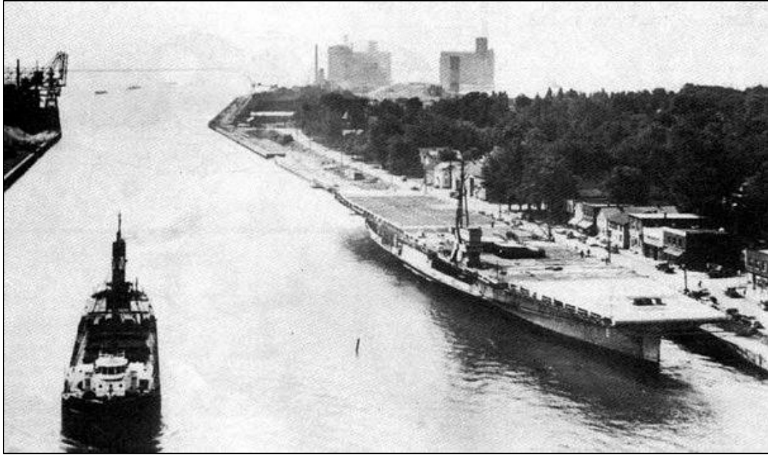
Figure 5.1. USS Sable passes the Welland Canal after being “shaved” (Courtesy, Warbird Information Exchange).
