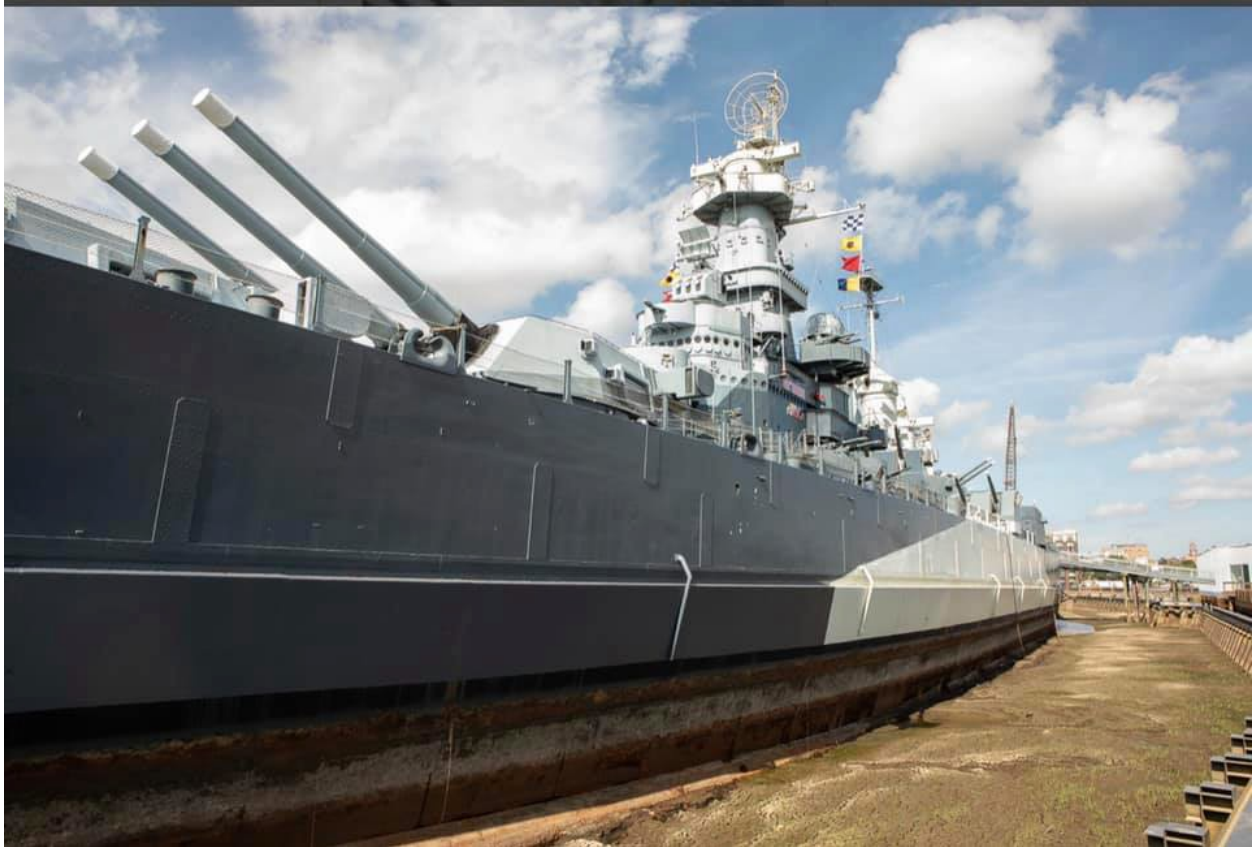
Figure 42. Image showing port side of USS North Carolina in a fully drained cofferdam. (Image by Joe Hollifield 2020)
