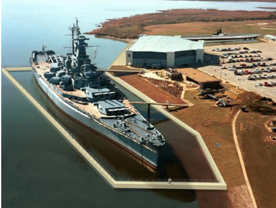
Figure 35. Image of permanent cofferdam installed around USS Alabama . Image from Amy Hotz 2010.
