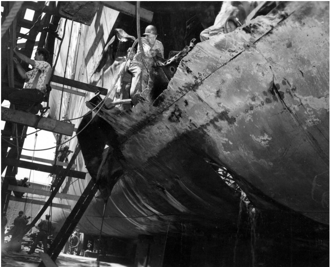
Figure 43. Workers at Pearl Harbor repairing damage to USS North Carolina suffered by a Japanese torpedo. (Battleship Memorial Archives 2019)
