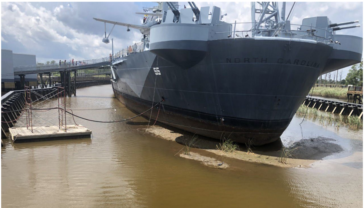
Figure 37. Stern view of USS North Carolina and cofferdam. (Image by Author 2020)
