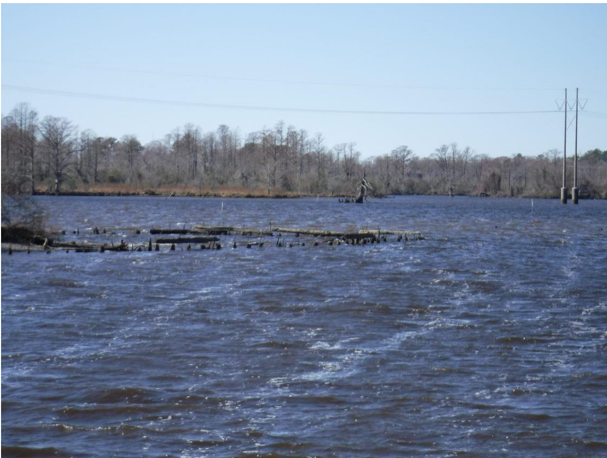
FIGURE 99. Western extent of log pool, showing horizontal beams secured to pilings by fasteners. (Photo by Will Nassif, February 2020)
