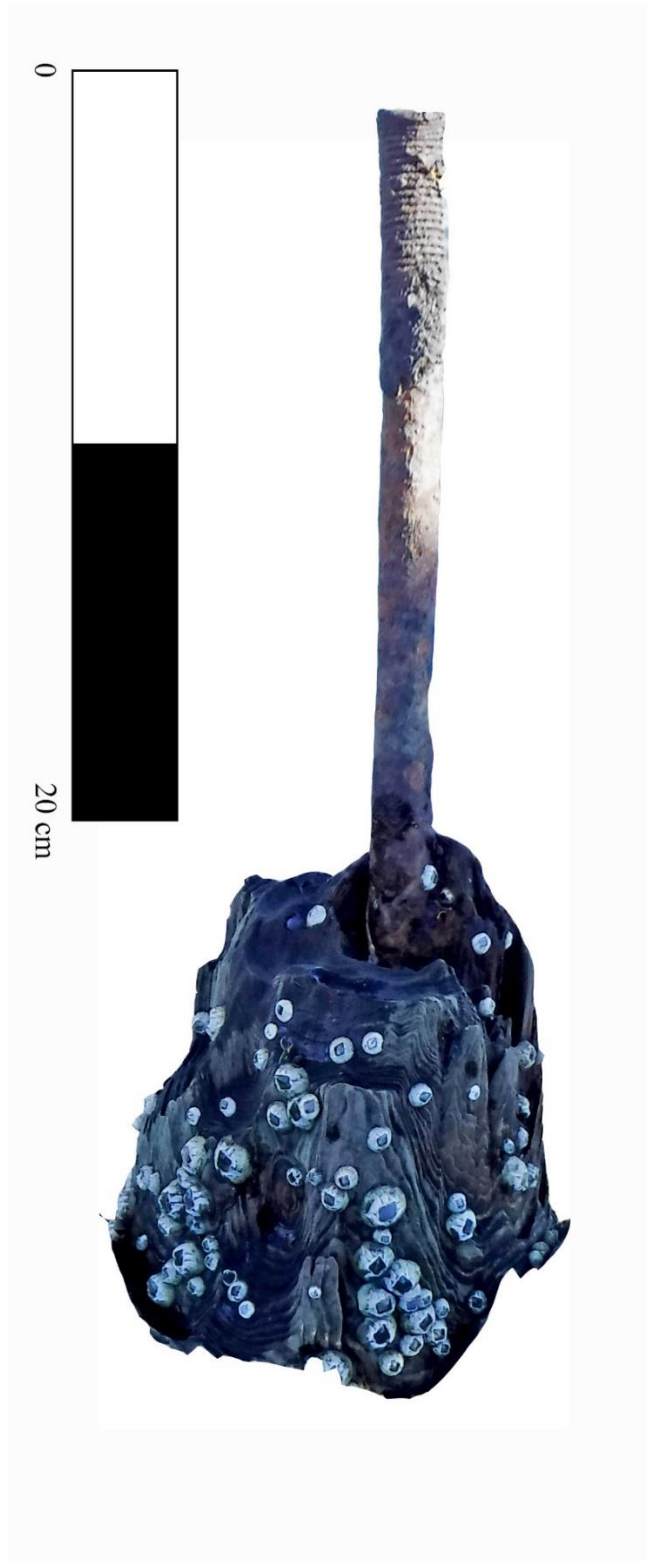
FIGURE 80. Piling and fastener from eastern pilings at Site B. (Photo by Will Nassif, February 2020)
