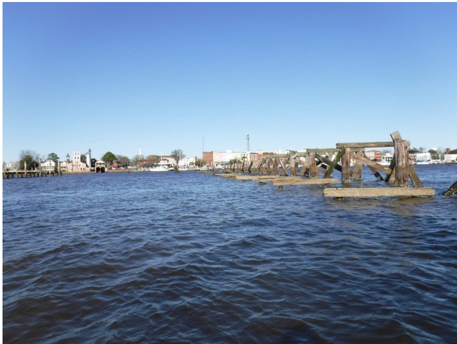
FIGURE 76. Eastern pier structure at S.R. Fowle & Son Company Sawmill. (Photo by Will Nassif, February 2020)
