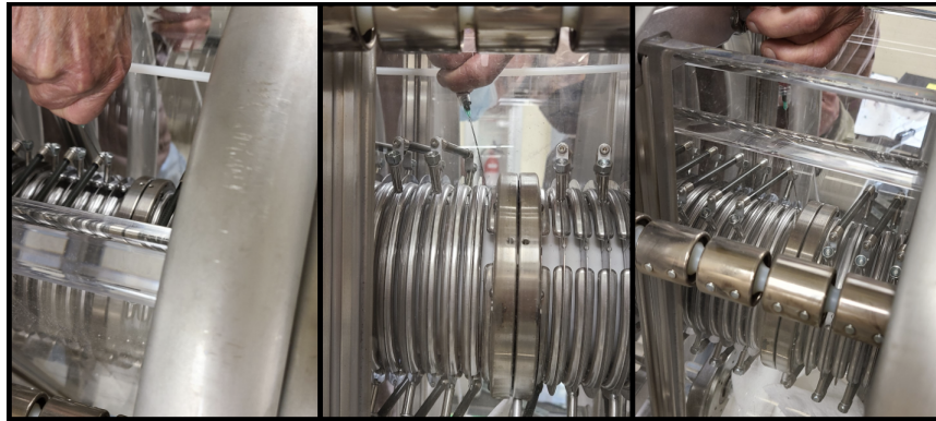
Figure 1.4: Each panel depicts the introduction/placement of the Glyptal paint which was used to seal the leak on the HE line.
