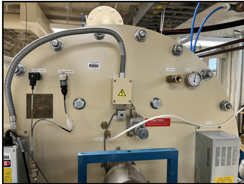
Figure 1.2: Shows the panel of the accelerator tank on the HE side that had to be removed to separate the tank from the beam line tube.
