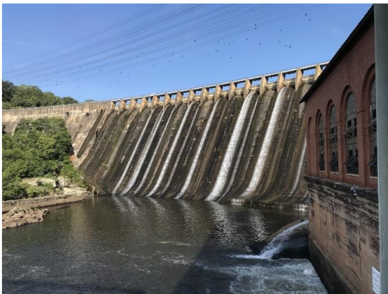
Figure 27. Narrows Dam and hydro station (Photo by P. Smith).
