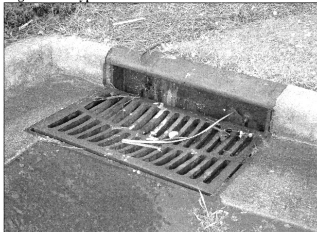
Figure 1-1: Typical curb inlet
