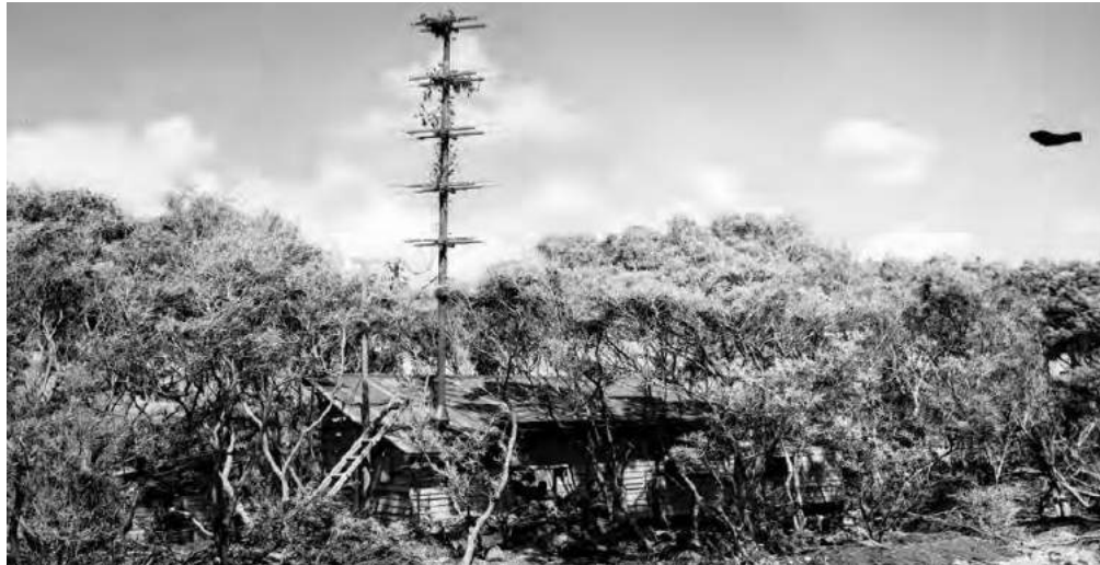
Figure 85. Type Mark 1 Model 3 Japanese search radar, Saipan 1944, 1300 yds. north of the eastern end of Aslito Airfield 1945 (Division of Naval Intelligence 1945).
