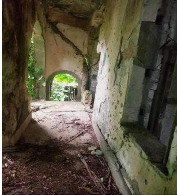
Figure 60. Japanese two-story Radar Hill headquarters, 2nd floor walkway (Photograph taken by author March 2022).
