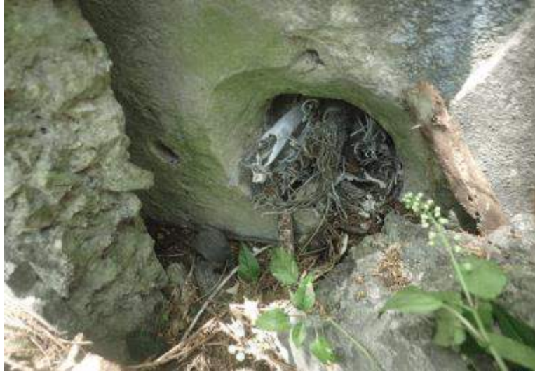
Figure 82. Naftan Peninsula radar emplacement building underground cable port with wires (Photograph taken by author 3 May 2023, no scale, facing east).
