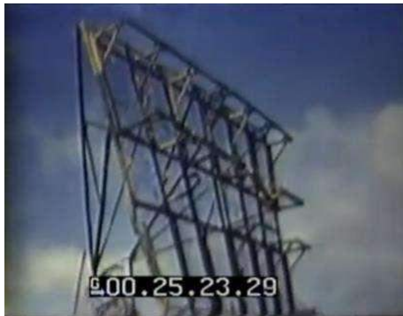
Figure 52. Japanese Mark 1 Model 1 aerial search radar on Radar Hill shown on post-battle footage (National Archives and Records Administration 1944c).
