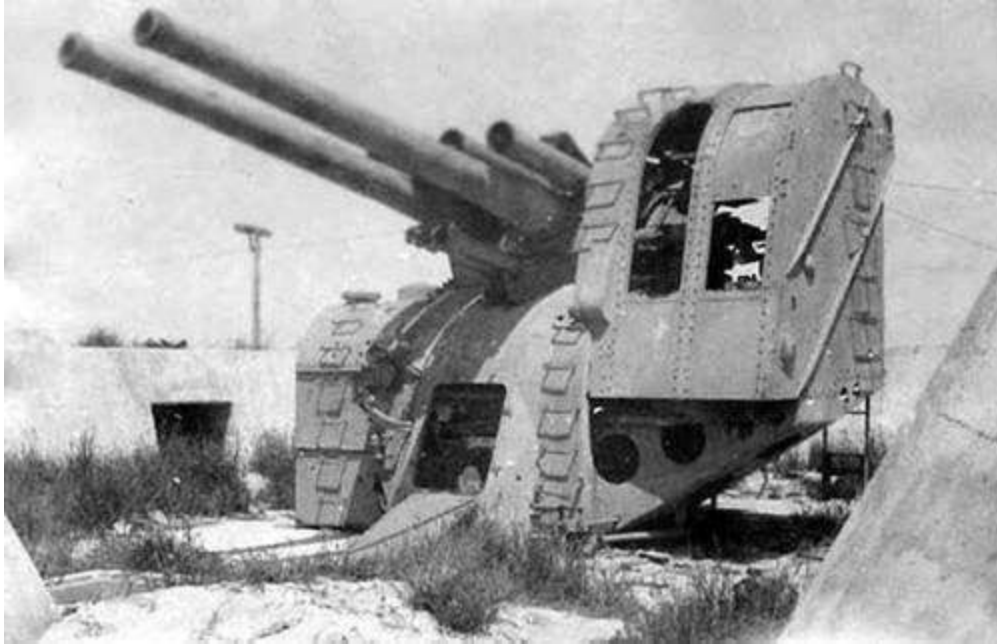
Figure 24. 127 mm. Type 89 dual-purpose AA and artillery gun (Office of the Chief of Naval Operations 1945b).
