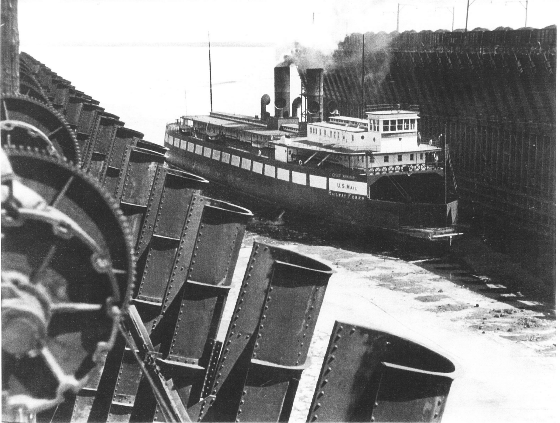
Figure 5. "Opening Escanaba." Chief Wawatam breaking open North Side of Dock #6 in Escanaba, Michigan. (April 10, 1937). Photo Courtesy of Great Lakes Marine Collection of the Milwaukee Public Library.
