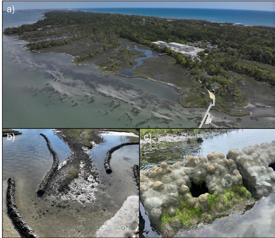
Figure 2. Aerial photo collected at 75 m from sUAS of TRNA Shoreline, Bogue Banks Barrier Island, Bogue Sound, and Atlantic Ocean (a). Example of Natrx ExoForms™ shoreline configuration and gap design captured from sUAS imagery (b) and structure design from ground image.
