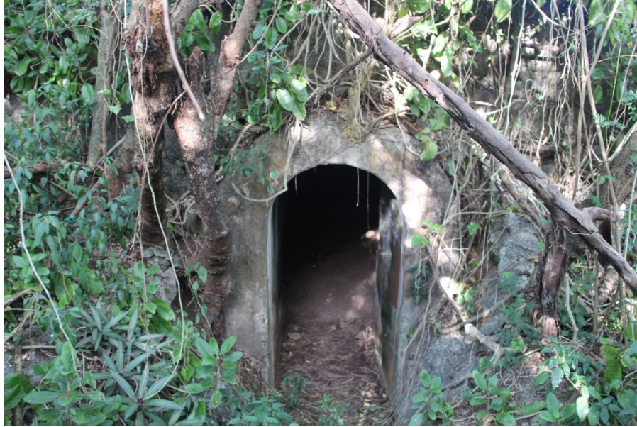
Figure 27: Entrance to Japanese gun emplacement overlooking Magicienne Bay, Saipan (Photograph by Author)
