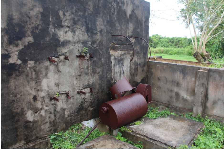
Figure 3: Air dryer in oxygen plant, Isley Field, Saipan (Photograph by Author)
