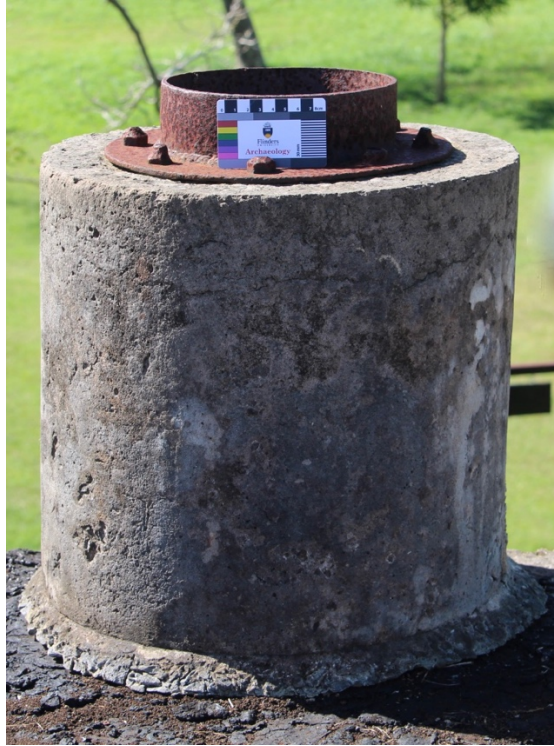
Figure 11: Chimney on bomb magazine, Isley Field, Saipan (Photograph by Author)
