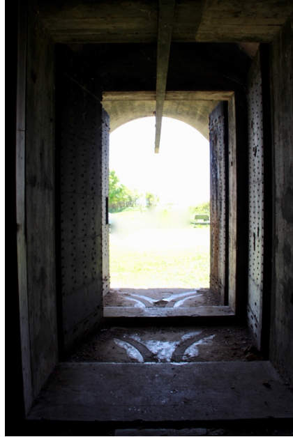
Figure 7: View of entry to bomb magazine from interior showing metal tracks in floor to open and close heavy double steel doors, Isley Field, Saipan (Photograph by Author)
