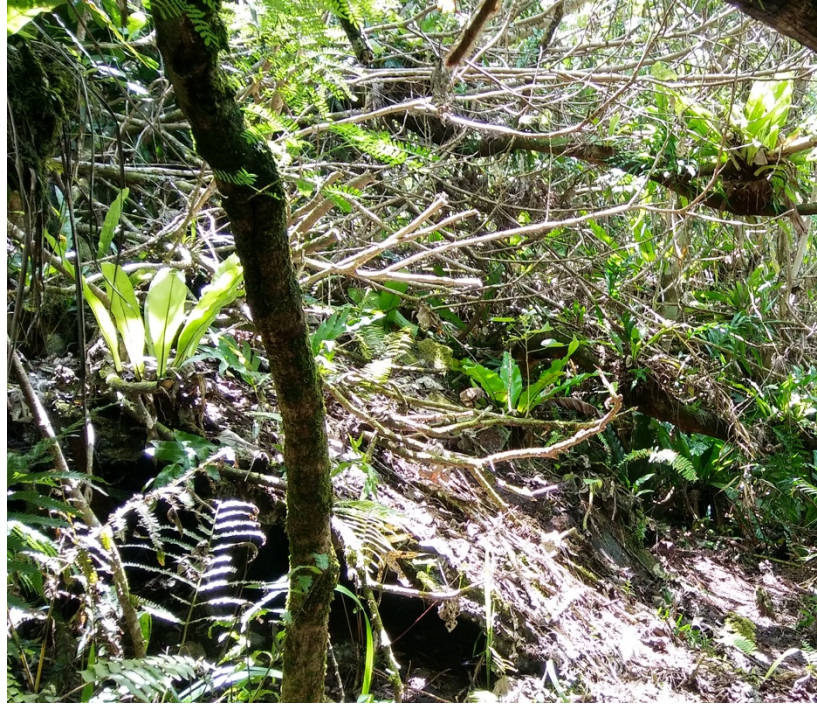
Figure 34: Photograph showing heavily overgrown wing section at the Jungle Site (Photograph by Peter Harvey)
