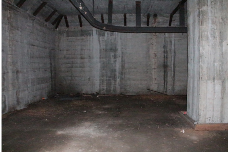
Figure 9: Interior of bomb magazine showing metal tracks used to transport bombs within magazine, as well as concrete pillars used to support reinforced ceiling, Isley Field, Saipan (Photograph by Author)
