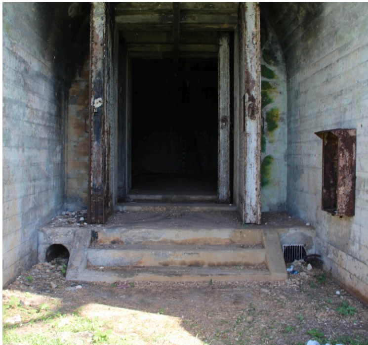
Figure 8: Entry to bomb magazine with still-visible camouflage paint, Isley Field, Saipan (Photograph by Author)
