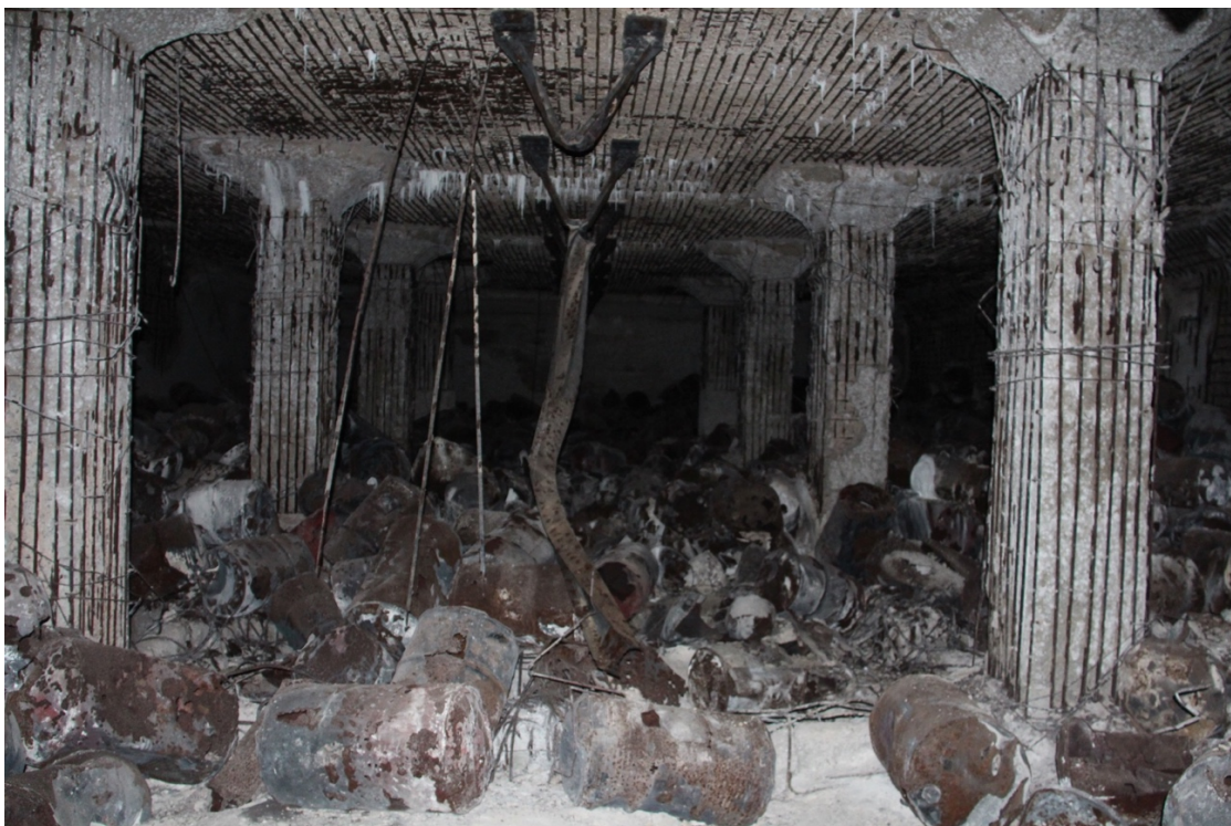
Figure 37: Japanese fuel Storage Facility interior showing damage from fire, North Field, Tinian (Photograph by Author)
