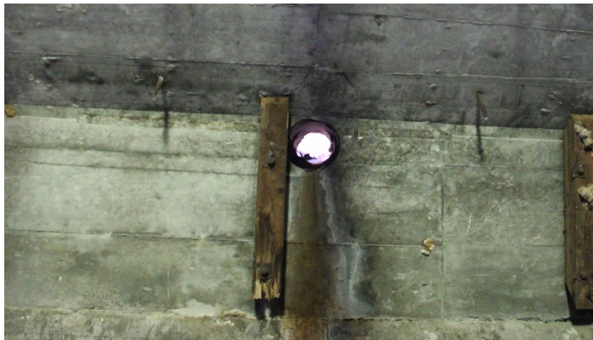
Figure 10: Chimney vent from inside of bomb storage magazine, Isley Field, Saipan (Photograph by Author)
