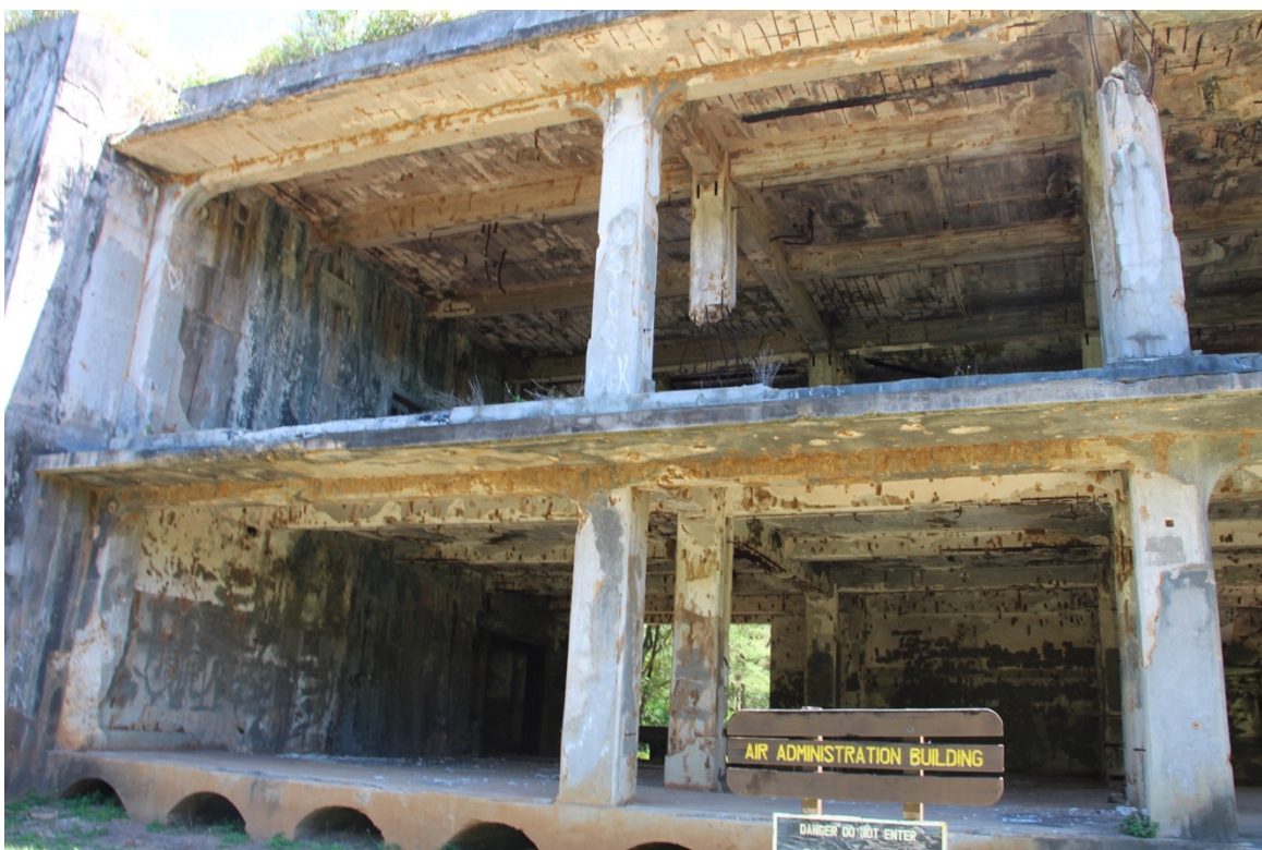
Figure 26: Japanese air administration building, Tinian (Photograph by Author)
