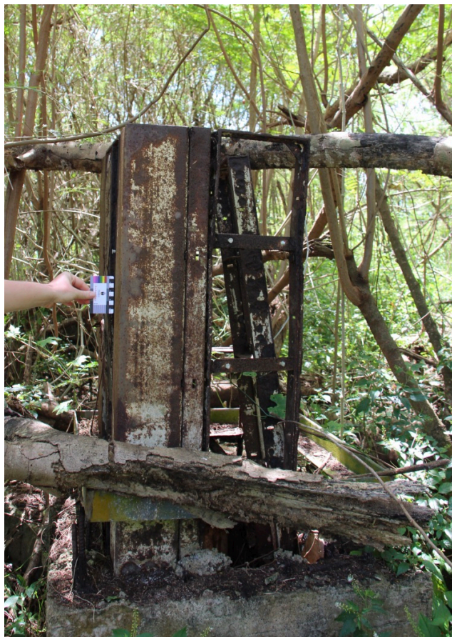
Figure 14: Well structure near railroad tracks, Isley Field, Saipan (Photograph by Author)
