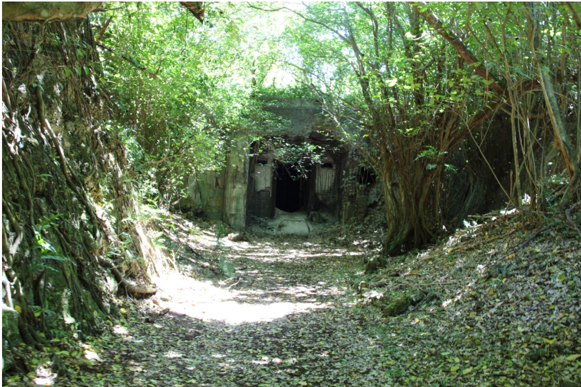
Figure 36: Japanese fuel storage facility, North Field, Tinian (Photograph by Author)
