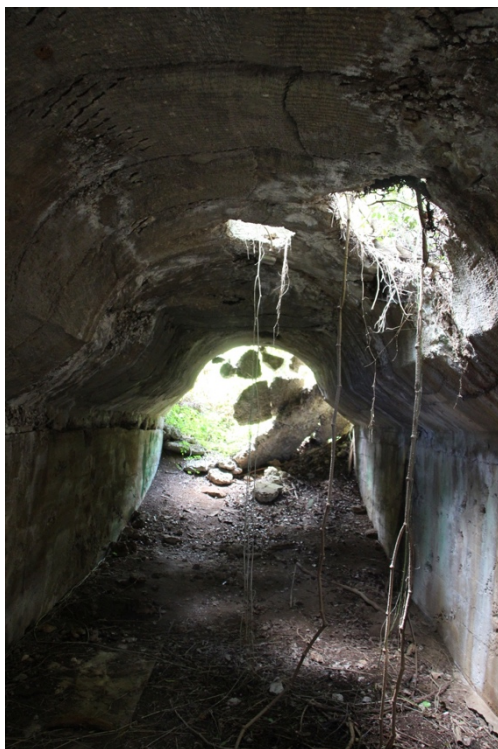
Figure 21: Japanese military storage facility, Saipan (Photograph by Author)
