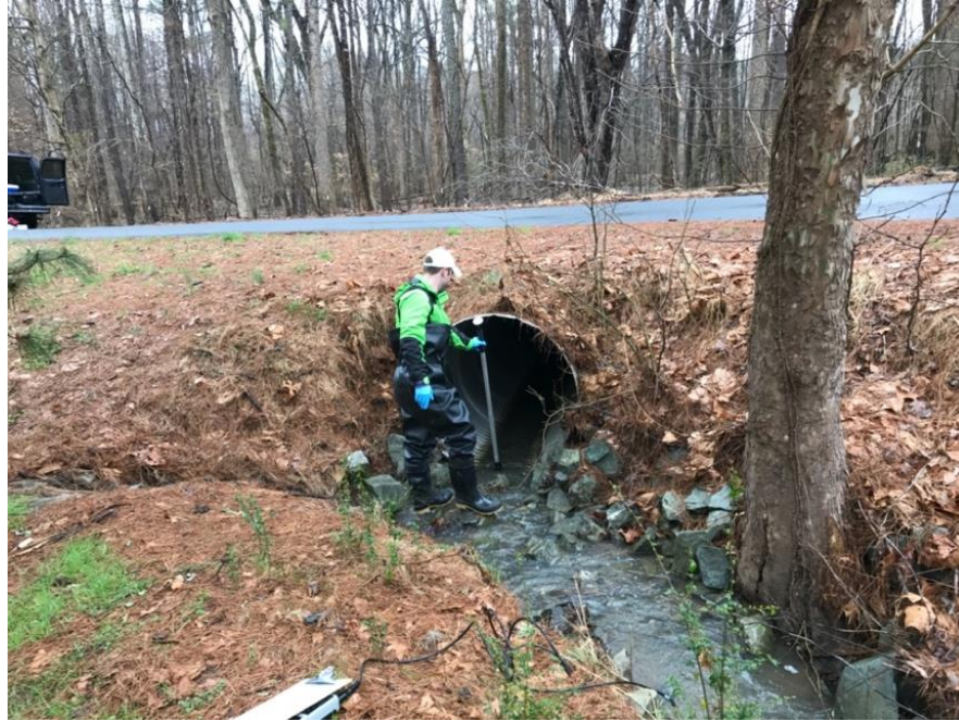
Figure 4A. Taking measurements at I-2 during baseflow.
