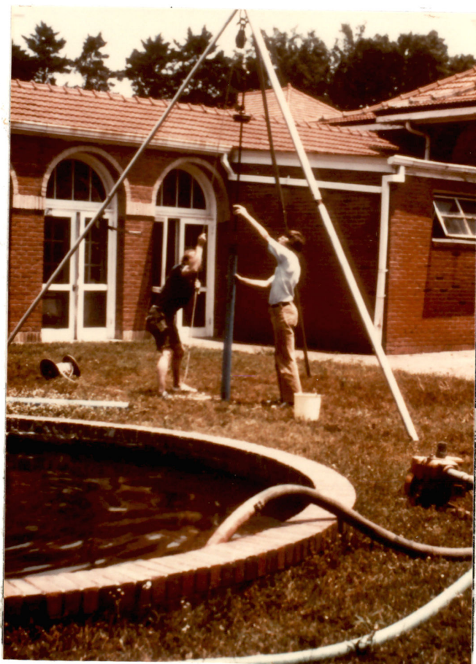
Figure 4: Photograph of coring equipment.
