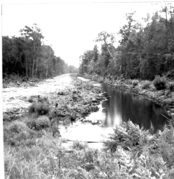
Second stage drainage ditch in Chowan County
