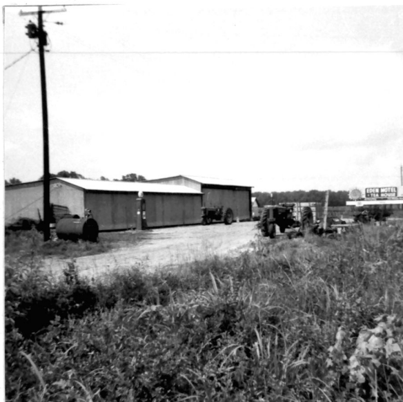
Equipment storage facilities, Perquimans County
