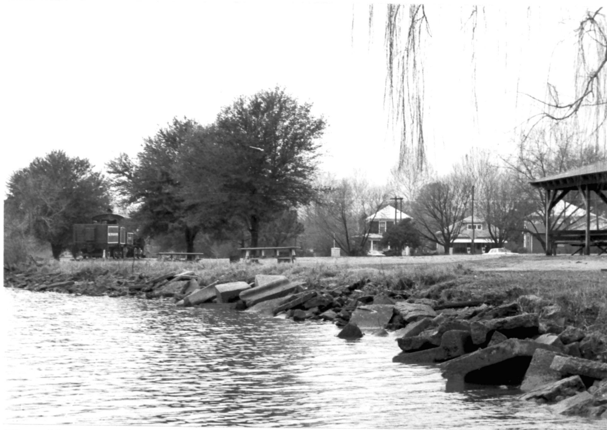
Fig. 23. Haven's Garden, public recreation land use on northern shore. It is a Type II shoreline with concrete rip-rap used to deter erosion.
