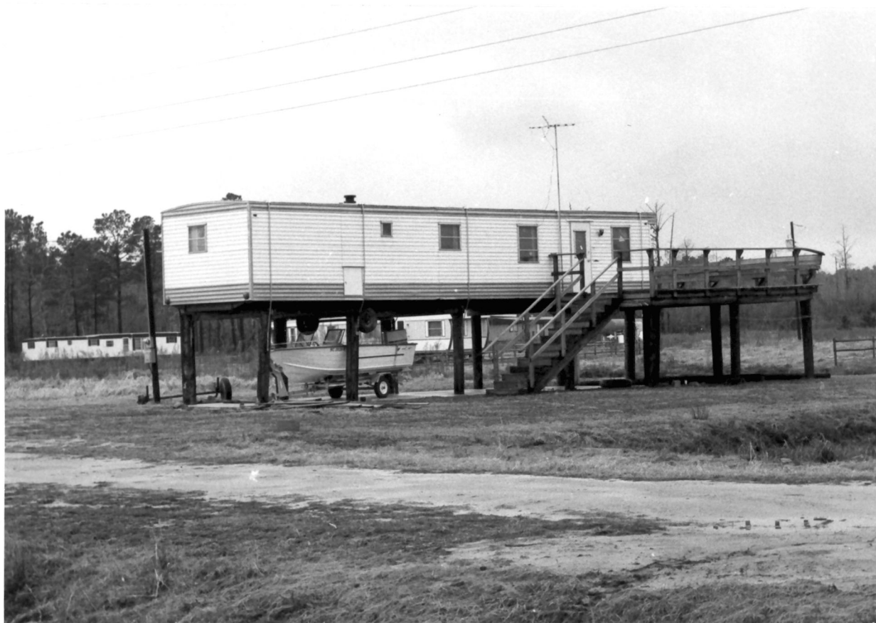
Fig. 26. Mobile home mounted on pilings, located on south shore near Whichard's Beach. It is along a former Type I shoreline, which has been altered through dredge and fill operations.
