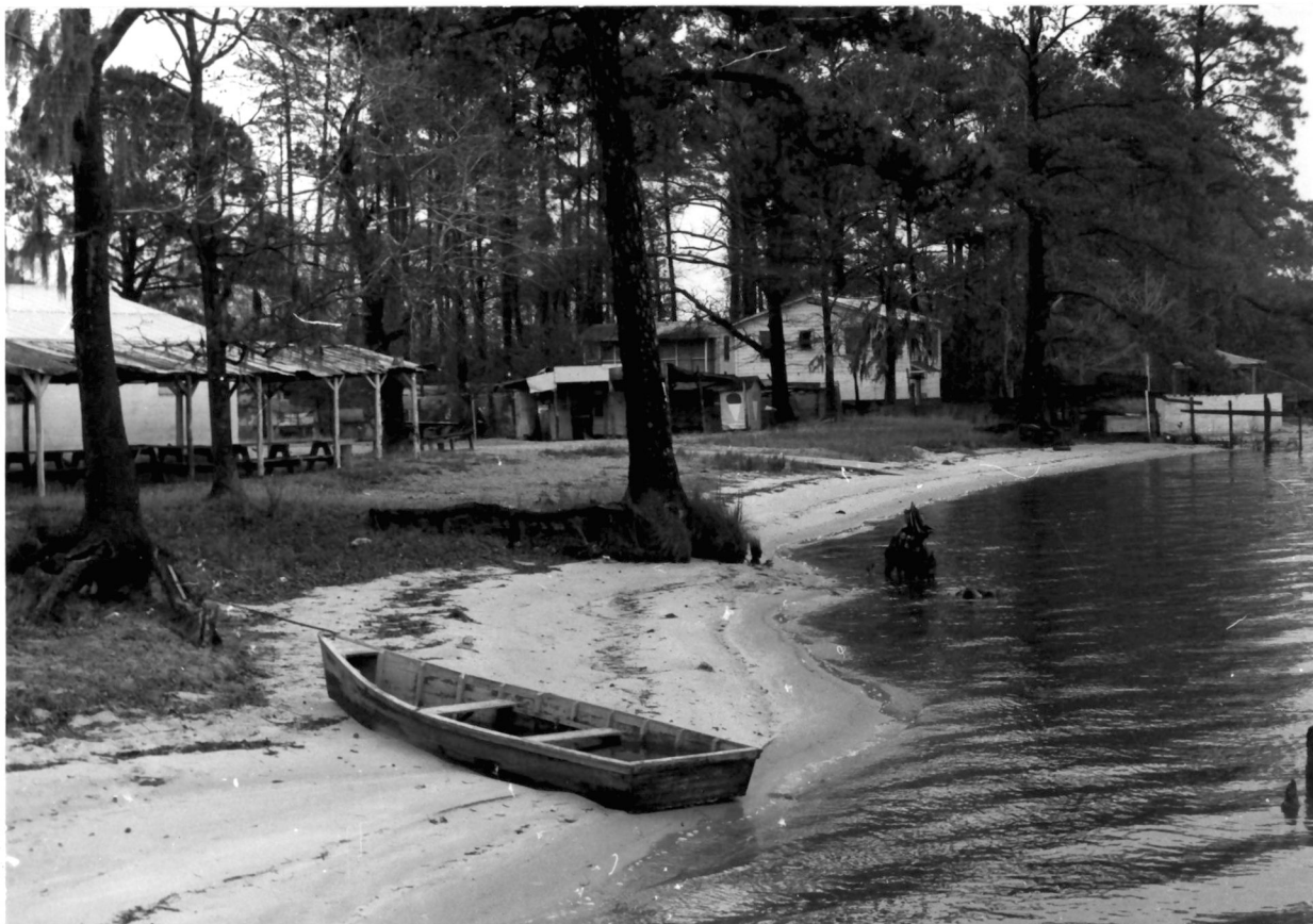
Fig. 24. Griffin's Beach, a Black commercial recreation area located on northern shore. It is a Type II shoreline experiencing some erosional activity as evidenced by the tree stumps offshore.
