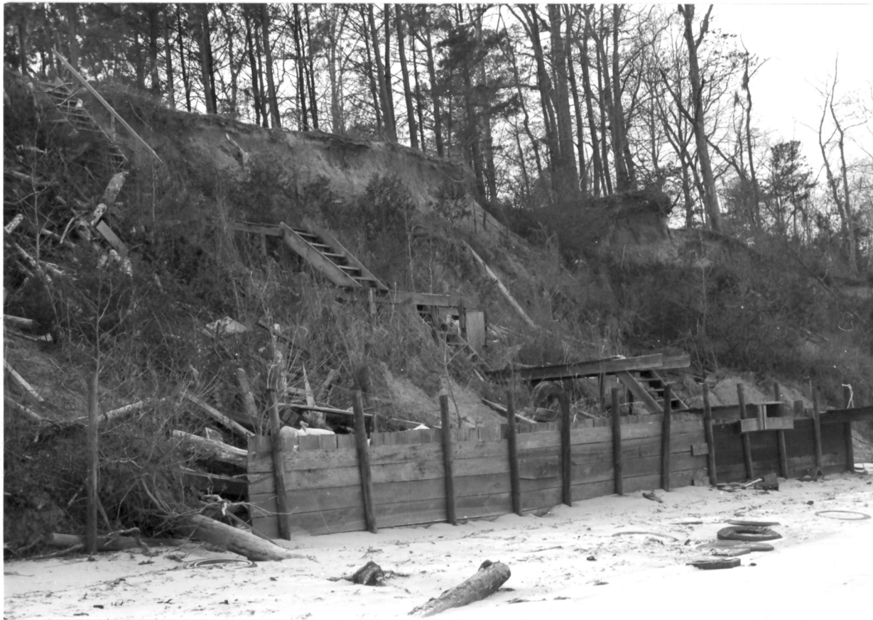
Fig. 15. Type IV shoreline located on south shore at Tripp Point. It is an area of active erosion. Residents have attempted to deter erosion by the use of bulkheads, tires, and assorted debris.
