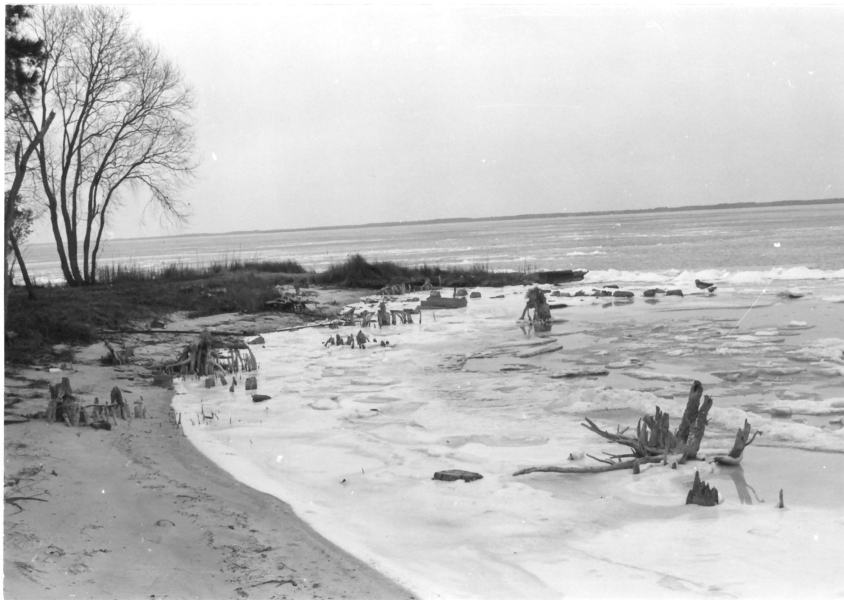
Fig. 20. Type II shoreline located on south shore near Hickory Point. Area of active erosion is indicated by the remnants of tree stumps in the water.
