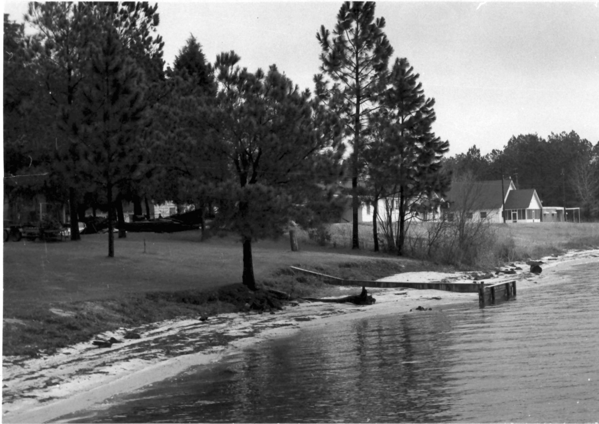
Fig. 25. Christian Service Camp, an example of institutional recreation located on the northern shore. Note the use of a groin to encourage deposition.
