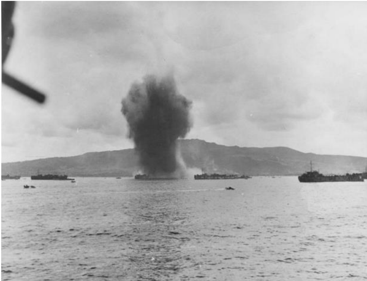
FIGURE B.7: UDT conducting explosive demolition operations on Saipan's barrier reef (Image courtesy NHHC).
