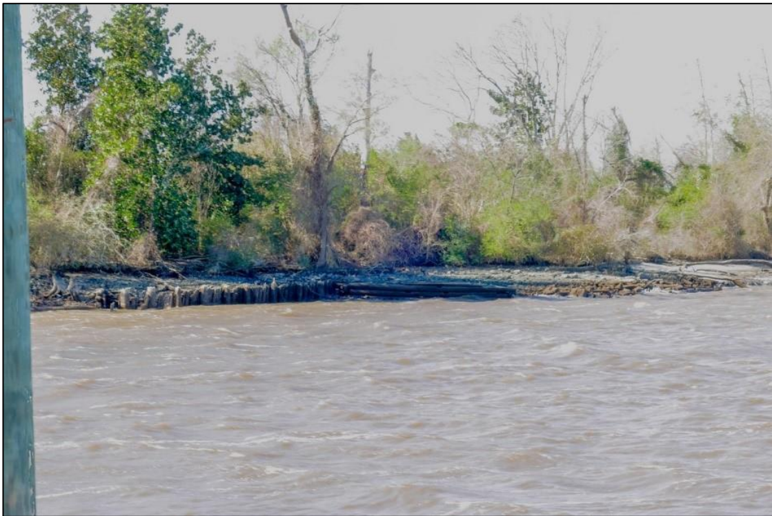
FIGURE 14: A closer examination of the wharf structure on the northern end of Castle Island. The cribbing timbers are exposed, as are ballast stones that were used to sink the cribs (Photo courtesy of Ray Midgett, 2021).
