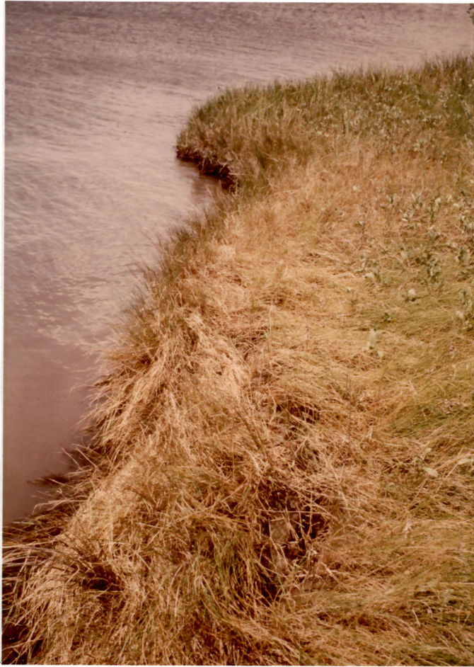
Figure 41. Cracks in the marsh surface root zone caused by the more rapid erosion of less resistant underlying peat.
