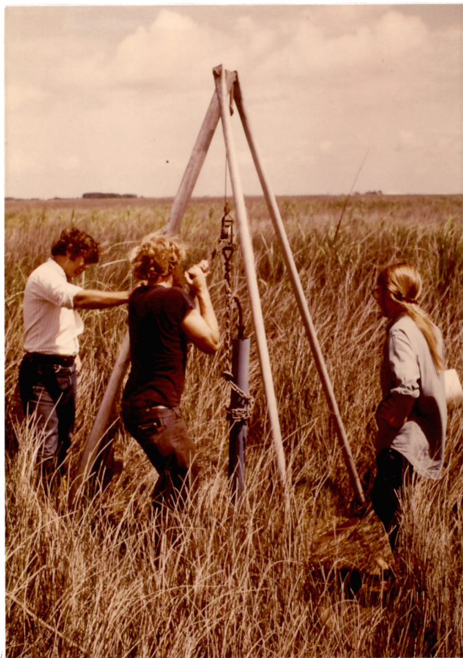
Figure 6. Removing a land core. Notice the plumers test plug sealing the top of the core barrel.
