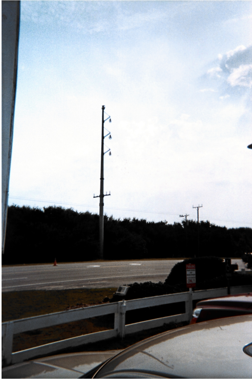
Figure 25: “The poles that they are putting up along the bypass are eyesores. I guess it will help to strengthen the utilities, but this is an ugly way of doing it.” - Paul
