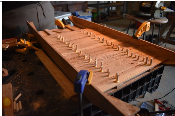
PHOTO 34. Photo showing treenails inserted into interior planking and stringers (Photo by Michaela Hoots).
