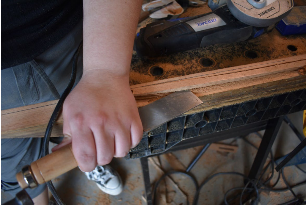
FIGURE 32. Photo showing carving technique used for the interior of the chine-girder (Image by Mark Newell).
