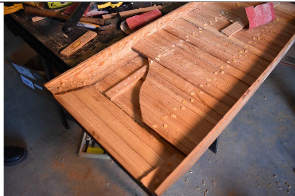
PHOTO 40. Photo showing the bottom interior planking, the ramp planking still unfinished (Photo by Michaela Hoots).
