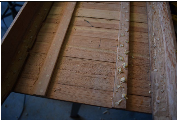
PHOTO 29. Photo showing difference between sanded treenails on stringers and unsanded (Photo by Michaela Hoots).
