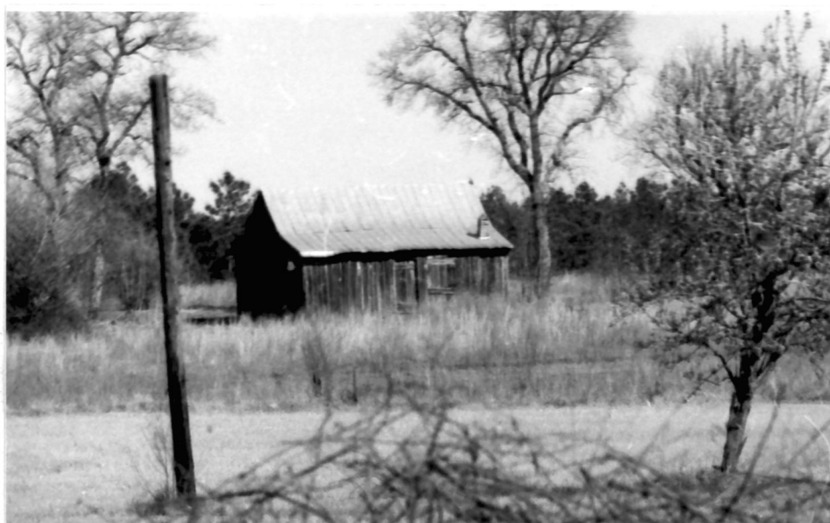
Fig. 15. Preserve Storage Building (Converted Dwelling)
