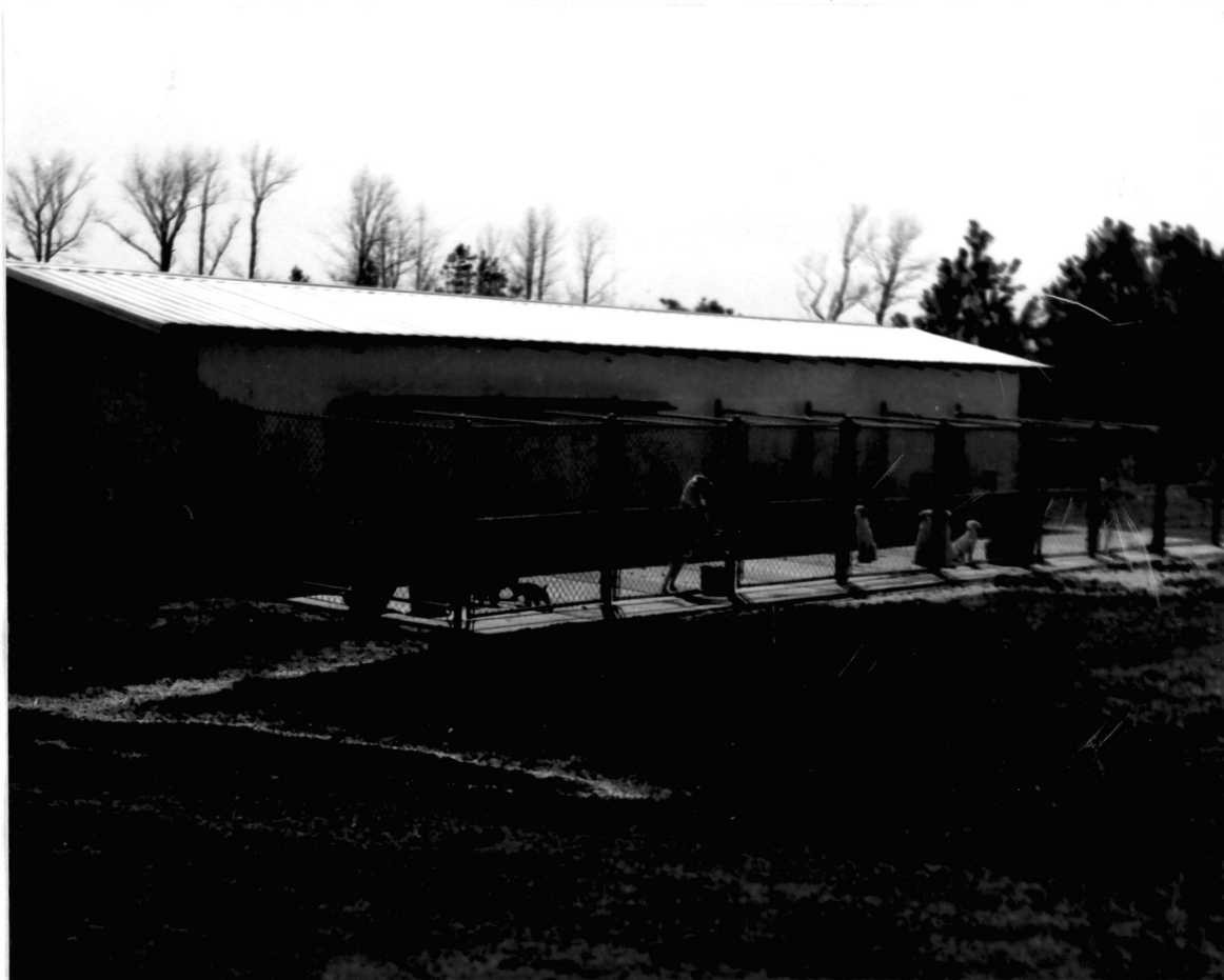
Fig. 13. Preserve Kennel - (Heated, Lighted)
