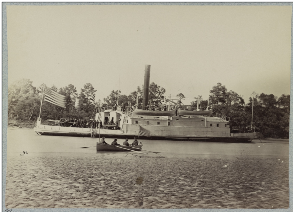
FIGURE 100. Photograph of vessel stated as Commodore Barney ; however, one can notice this is the same vessel as Figure 94. Note the acting stern end's low draught with water meeting the strut planking. This may have provided additional buoyancy (courtesy of the National Archives; reference # 2013647361).
