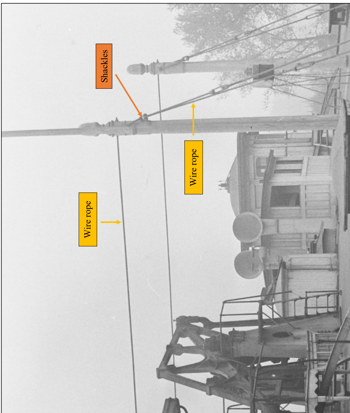
FIGURE 68. Hurricane deck of ferryboat Atlantic at East Kingston, New York, to be dismantled. Note shackles and wire rope connected to cross braces (courtesy of the Elwin Eldridge Collection, The Mariners Museum and Park Archives, Newport News, Virginia; reference # MS0091/03.01-04-061a).
