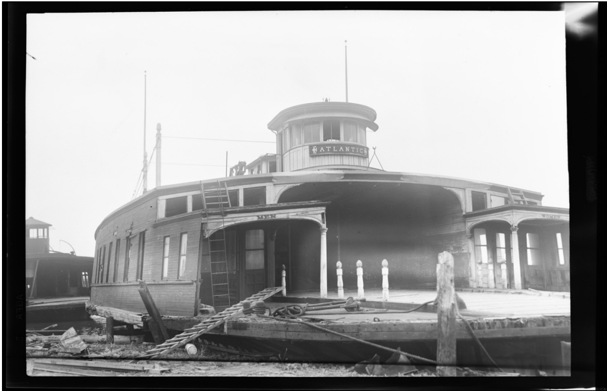
FIGURE 50. Main deck of New York ferryboat Atlantic (built 1884) at East Kingston, New York to be dismantled, 1939. Note the slight drooping of the deck as it continues outboard (courtesy of the Elwin Eldridge Collection, The Mariners Museum and Park Archives, Newport News, Virginia; reference # MS0091-03.01-04-061B).
