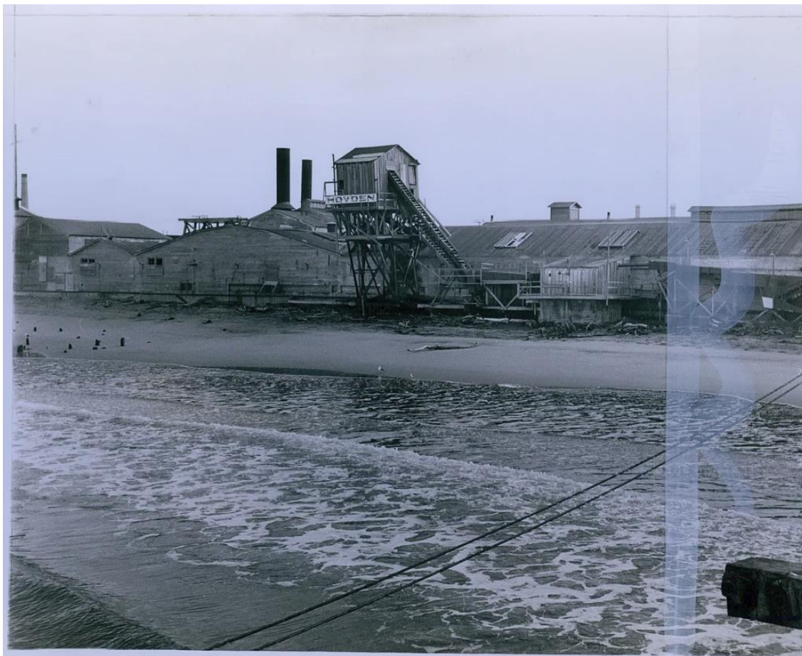
FIGURE 32: Historic photograph of Hovden Sea Foods, depicting the possible remains of slipway supports in the center-left. (Pat Hathaway Collection).
