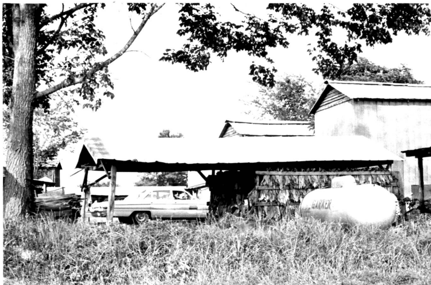
Figure 24.--Looping shelter with sheet metal roof
