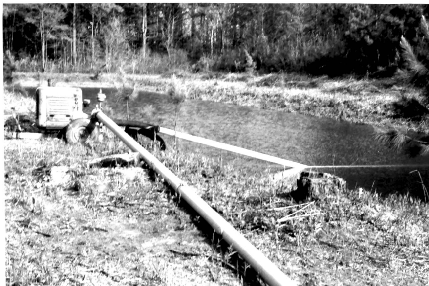
Figure 17.--Gasoline pumps draw water from irrigation pits.
