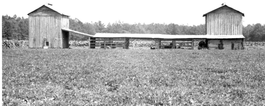
Figure 27.--Shelter extending between two barns
