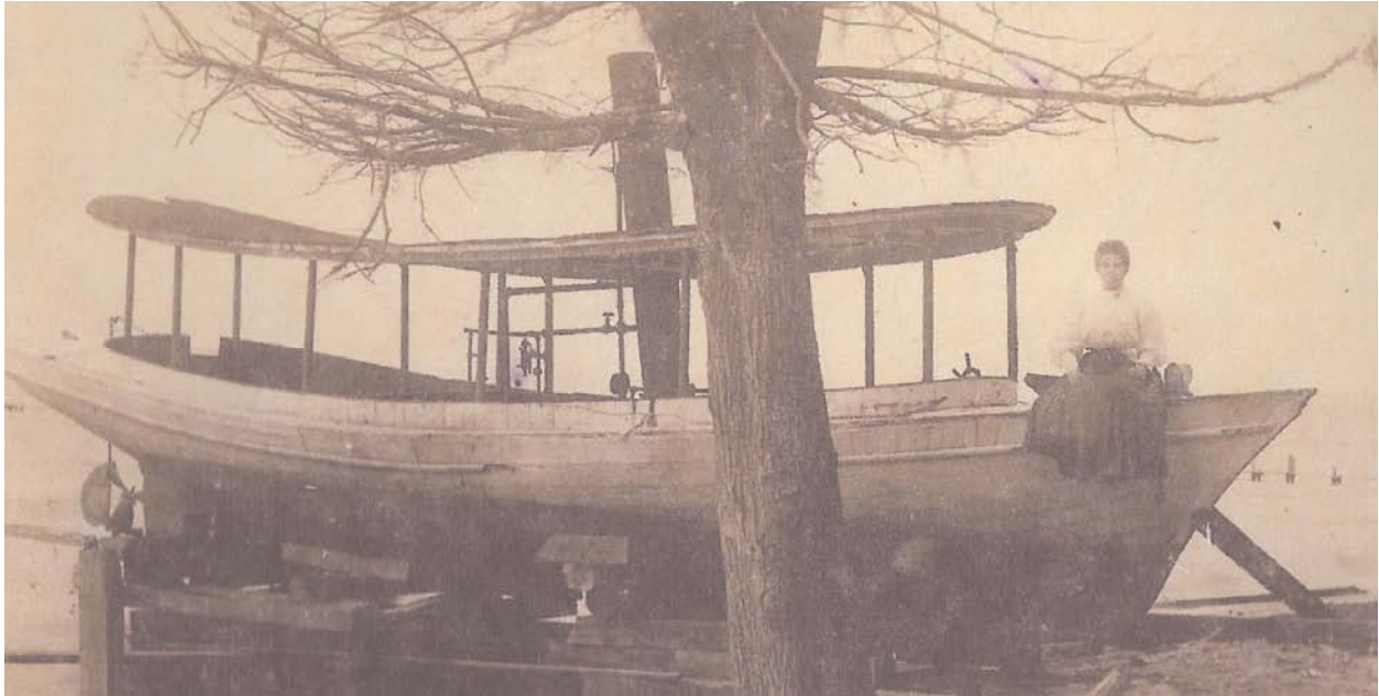
FIGURE 22: Mrs. Potts sitting on the Bohemian Girl . It is assumed this photograph was taken the same day as Figure 20. Note the steering wheel at the forward end of the cockpit, steam pressure gauge located directly aft of the smoke stack, and steering quadrant attached to the whipstaff (Photograph courtesy of the Lake Waccamaw Depot Museum).
