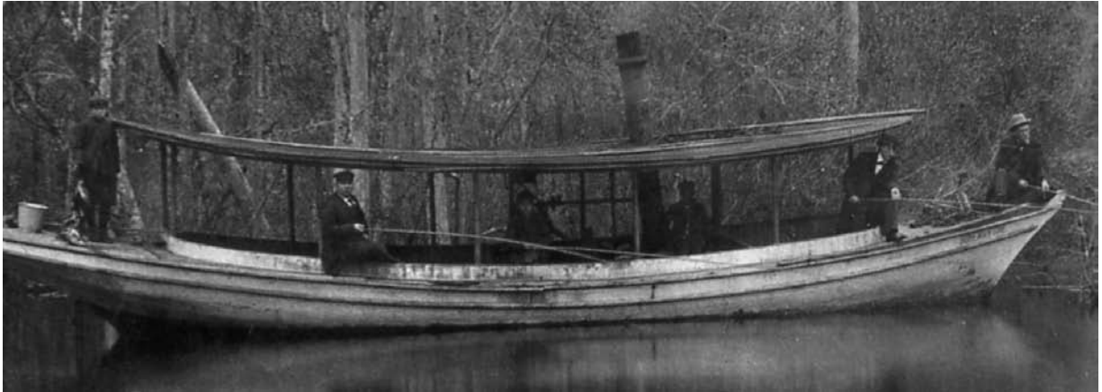
FIGURE 18: The Bohemian Girl in Big Creek. Note the smoke stack, no steam whistles, and two rub rails that were similar to the vessel depicted in Figure 16 (Photograph courtesy of the Lake Waccamaw Depot Museum).
