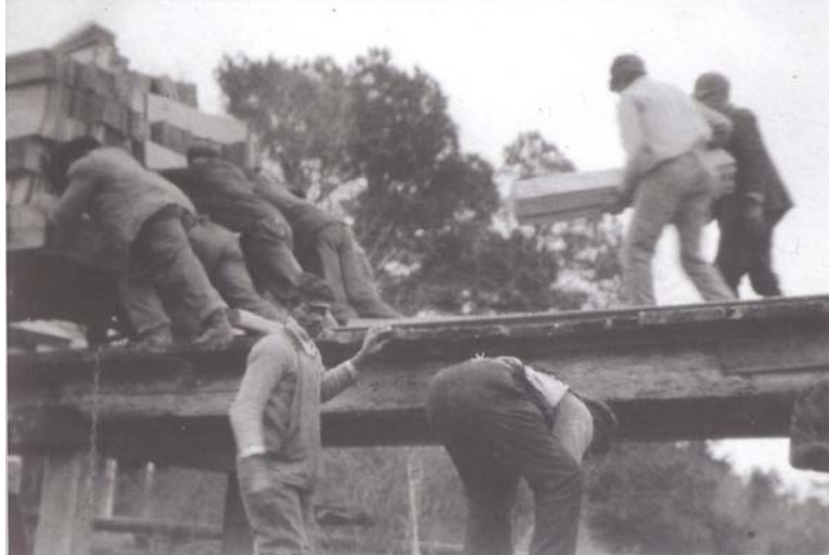
FIGURE 12: Laborers pushing a shingle load off the pier (Courtesy of the Lake Waccamaw Depot Museum).
