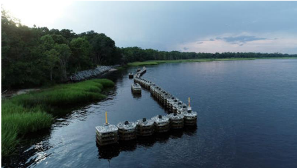
Figure 3.15 Wave attenuators and riprap near Battery A. (Image courtesy of Atlantic Reefmaker)
