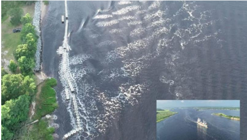
Figure 3.16 Attenuating waves at BTFA (Image courtesy of Atlantic Reefmaker)
