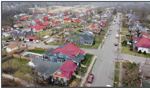
Figure 3: Drone Image Analysis Implementation to Identify Tarped Roofs
