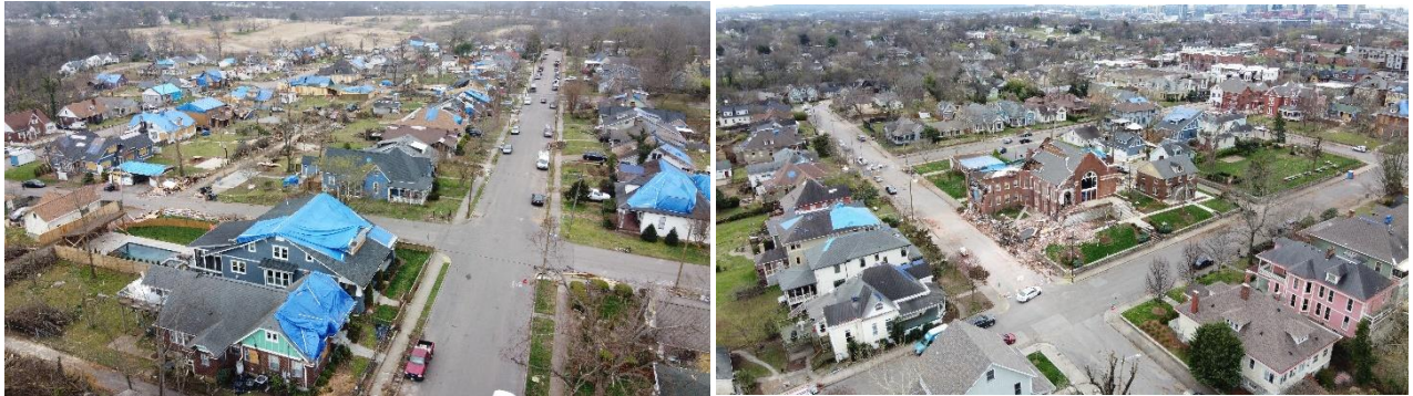
Figure 1: East Nashville Tornado Damage
